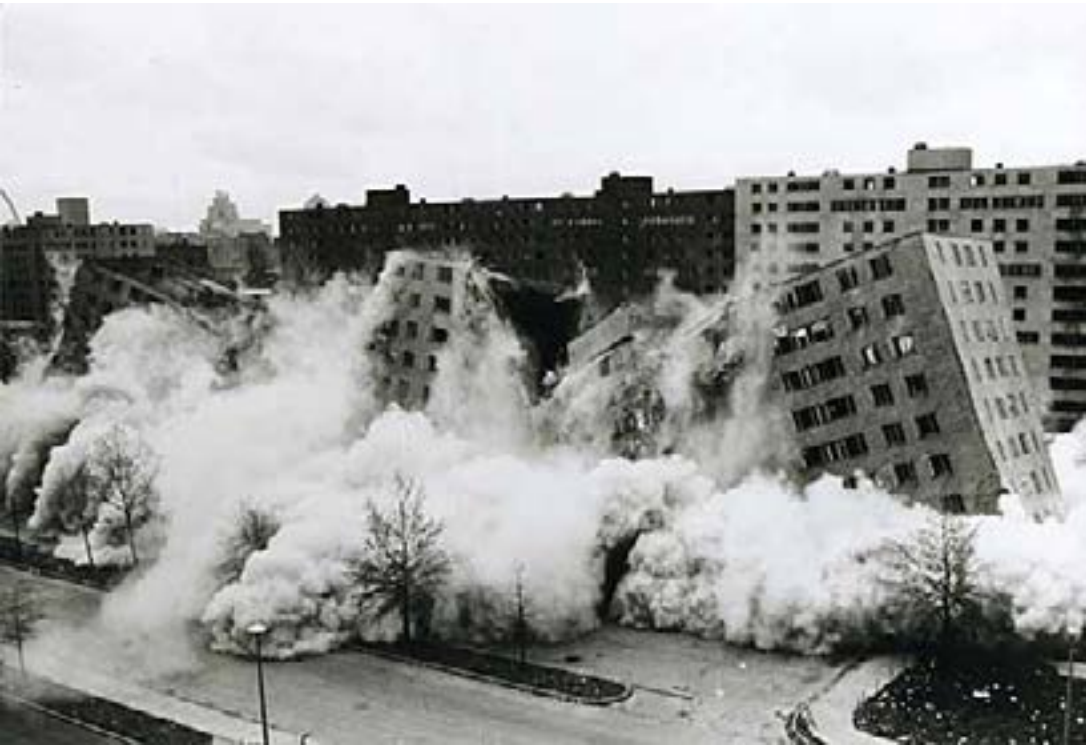
Pruitt-Igoe Housing Development
