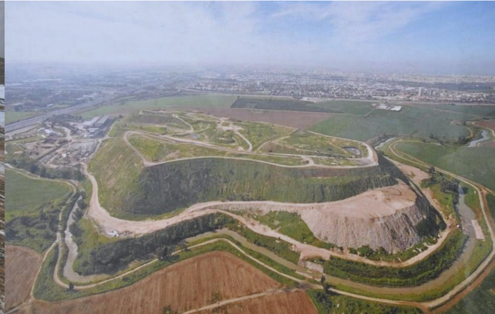
Wall prevents the collapse of the mountain
